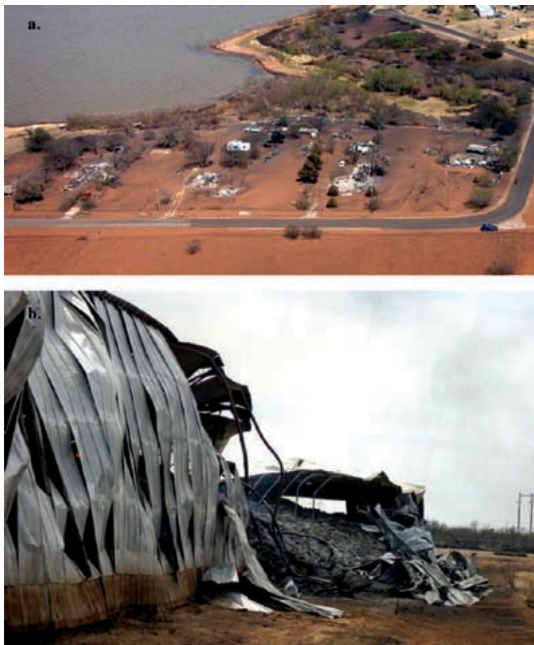
FIG. 1. (a) Home and property destruction near Archer City, TX. (b) Steel-framed storage barn destroyed near Electra, TX. Note that the heat of the fire has deformed the metal frame. Photographs courtesy of the 10 Apr 2009 edition of the Times-Record News of Wichita Falls, TX.
